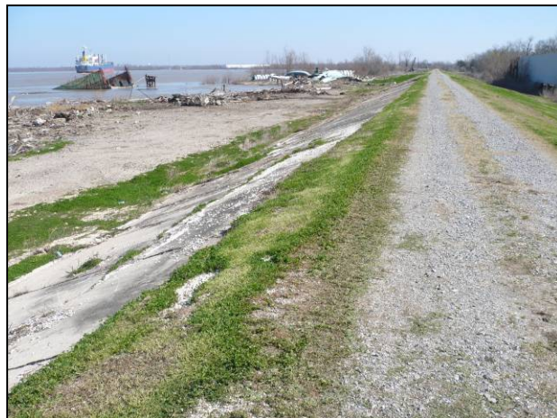
Figure 38: Bender Shipyard – Upstream Levee and Batture
