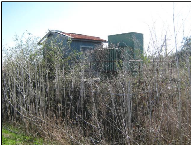
Figure 50: Bender Shipyard – Electric Transformer
