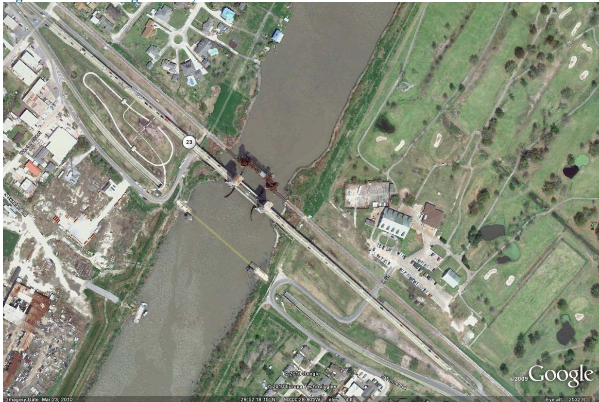
Figure 9: LA 23 Bridge/Tunnel, Belle Chasse
