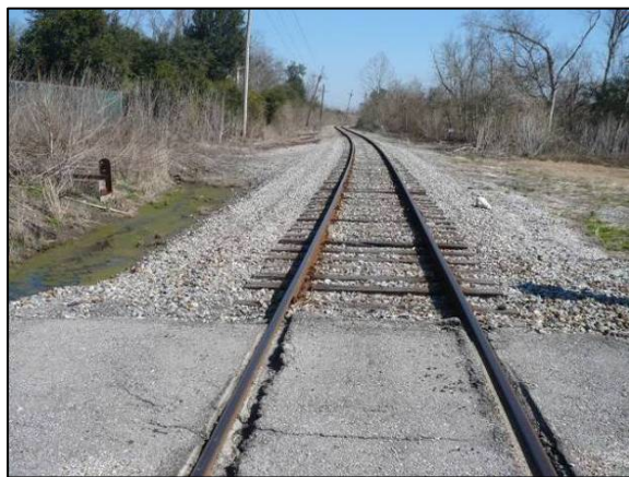
Figure 44: Bender Shipyard – NS Louisiana Southern Rail Line Approach
