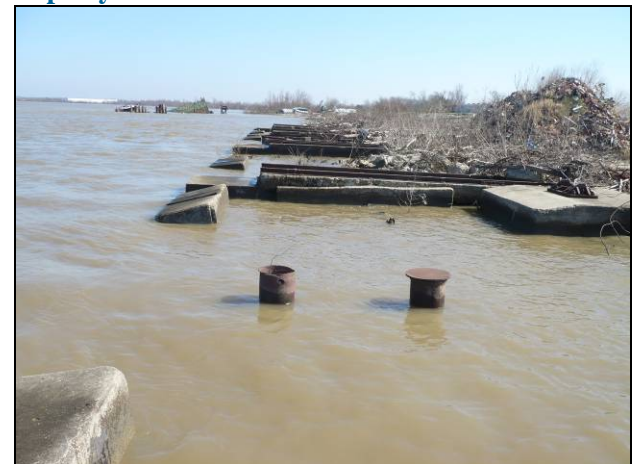
Figure 39: Bender Shipyard – Abandoned Slipways
