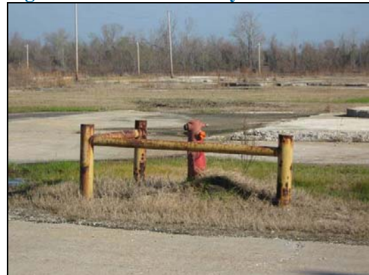
Figure 16: Amax – Fire Hydrant
