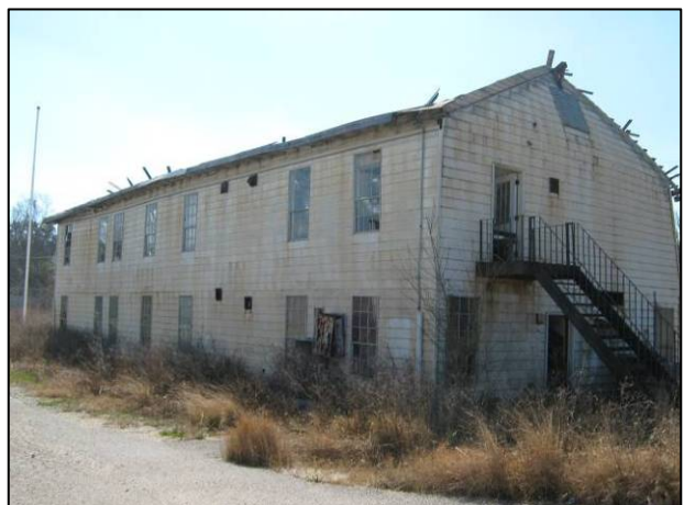
Figure 49: Bender Shipyard – Structure No. 5
