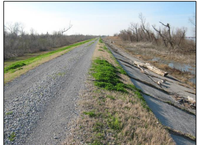
Figure 59: Citrus Port Site – Levee and Batcher
