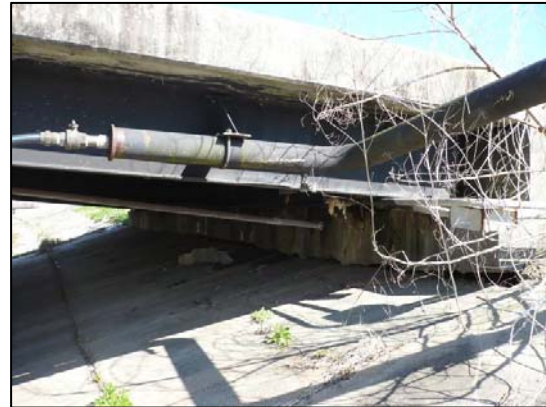
Figure 6: Amax – Pier Utility Connections
