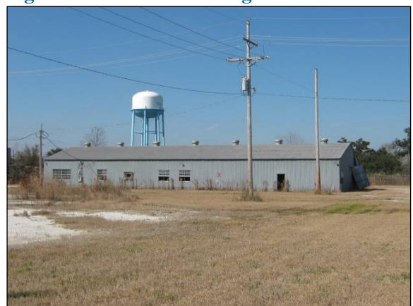
Figure 14: Amax – Building No. 4
