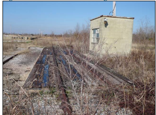
Figure 10: Amax - Rail Car Weight Station
