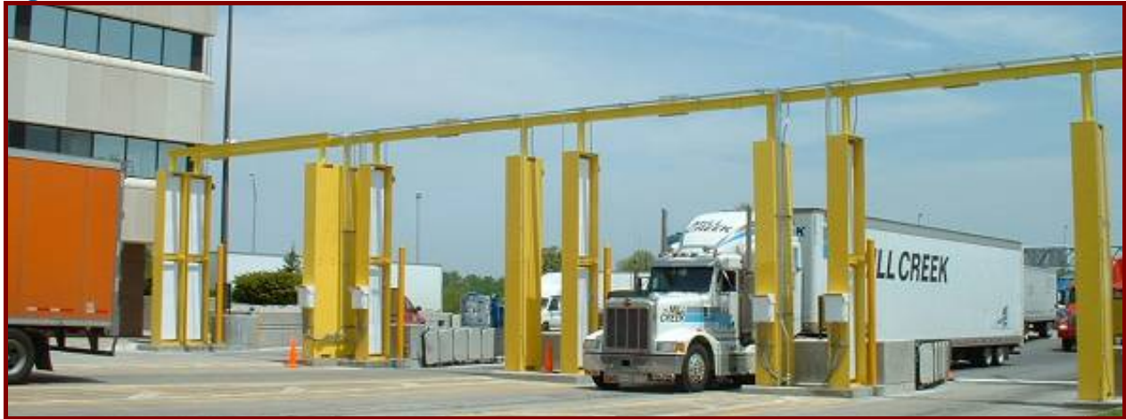
Figure 26: Portal Radiation Scanners
