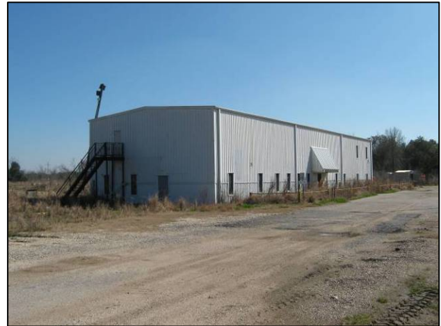
Figure 47: Bender Shipyard – Structure No. 4
