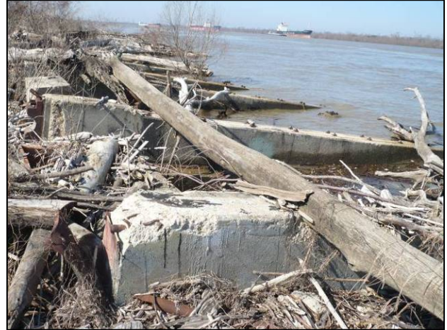
Figure 41: Bender Shipyard – Abandoned Slipways
